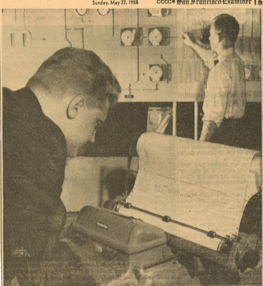
NEW - Bob Kohler, left, and Ed Jones demonstrate a highly advanced machine which automatically assembles information on a plant operation spread over many acres. Control panel in background keeps track of operations. Information is sent to high speed typewriter which makes record - in red if off normal condition is noted. This type of machine is important phase of automation, which promises new era in Nation's industry.
