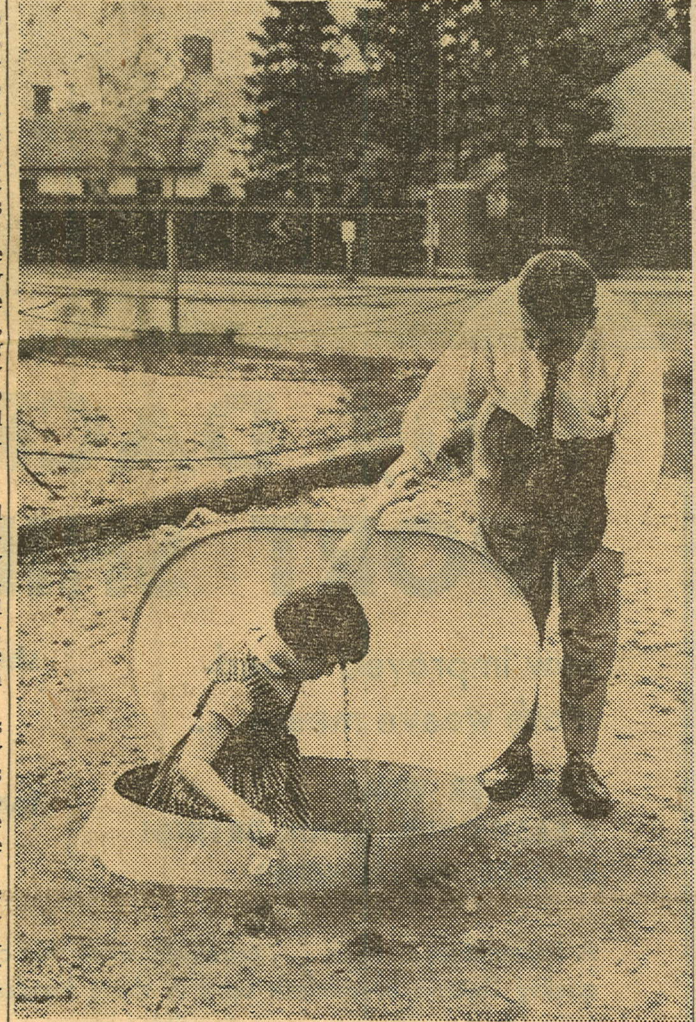
ENTRANCE —A youngster is helped into the hatch-like entrance to the Walter Kiddie Laboratories H-bomb shelter shown above. At right background is the intake for the special filter which removed radioactive particles from the air.
